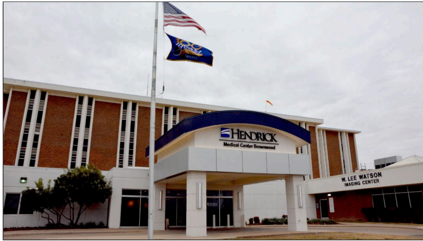
A new canopy at the Hendrick Medical Center Brownwood front entrance is one of many upgrades made to the facility since joining Hendrick Health in 2020.
